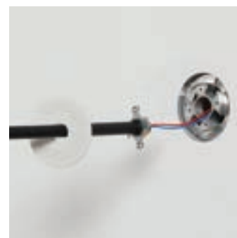
Connect fixture to junction box.
