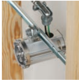
Connect power from conduit to junction box.
