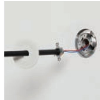
Connect fixture to junction box.
