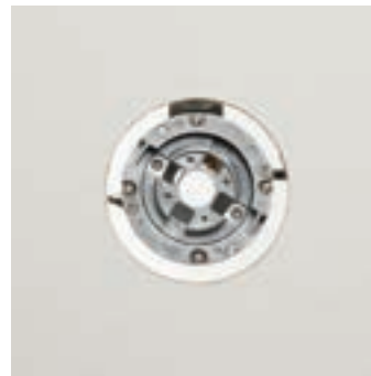
Install the drywall.
