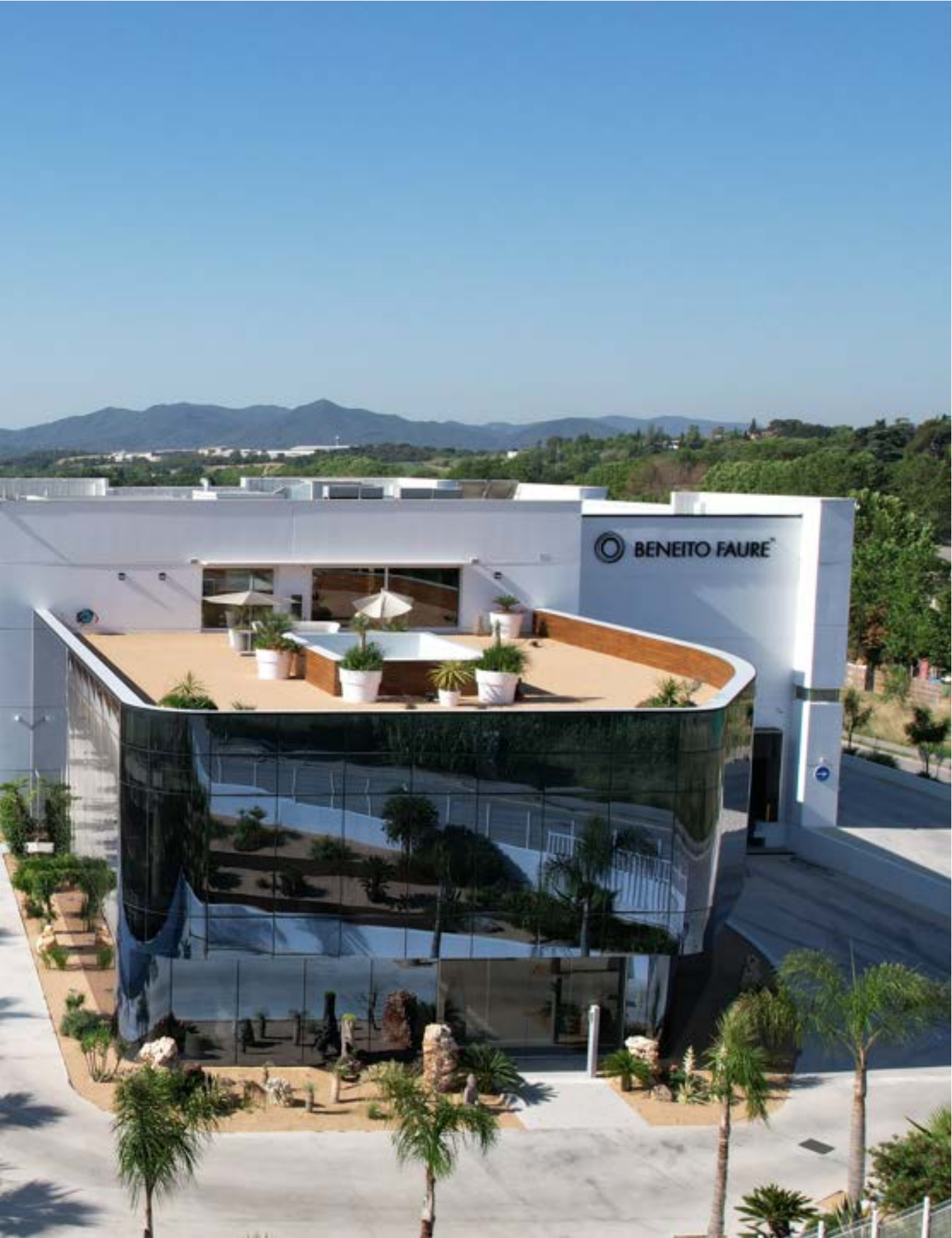
Showroom Beneito Faure, La Roca del Valles (Spain).
